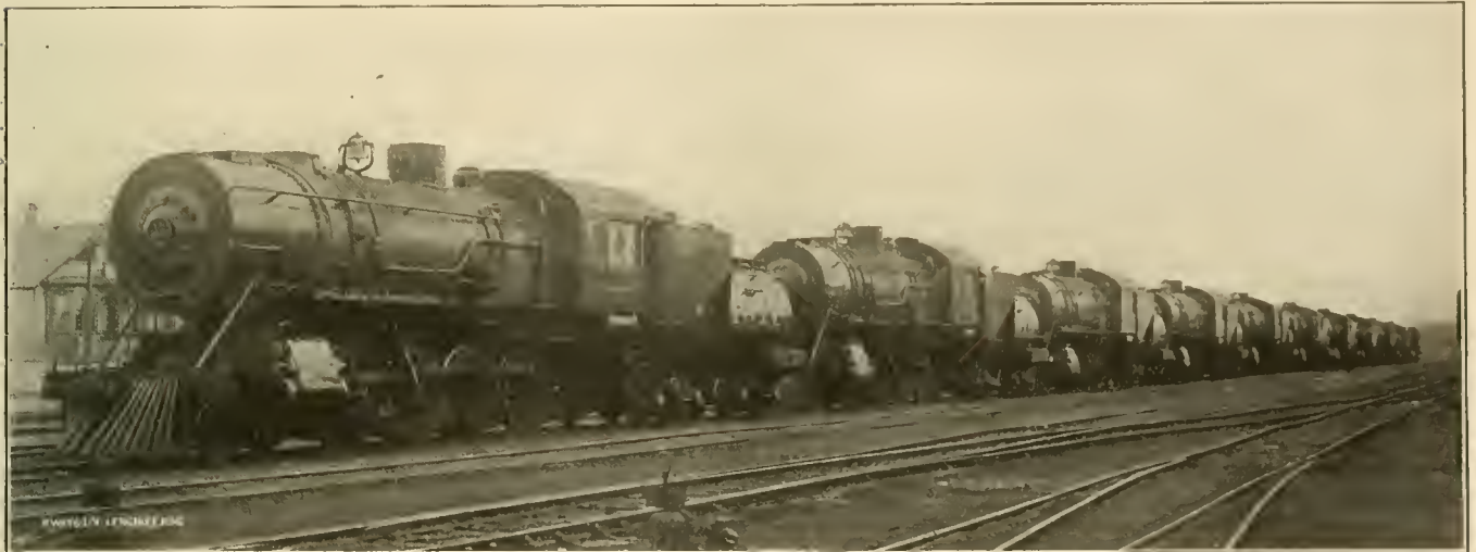
STRING OF CONSOLIDATIONS, WITH VANDERBILT TANKS, FOR THE OREGON SHORT LINE.
